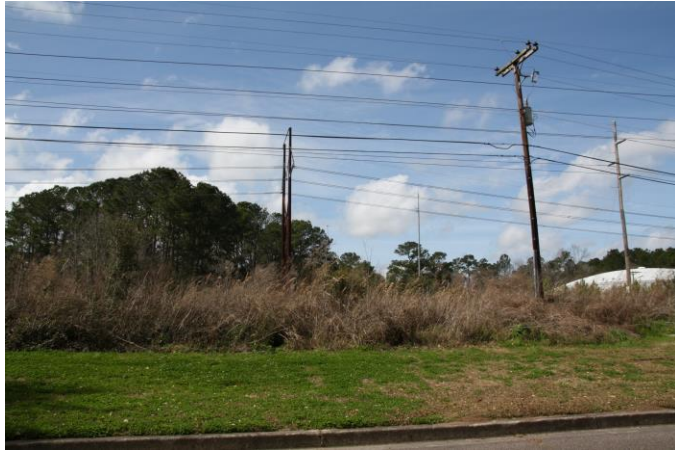
WEST – Undeveloped property adjacent to west of site Facing west from Shipley Street Power lines are in forefront of picture, Charleston DPW water pump station facility can be seen to right
